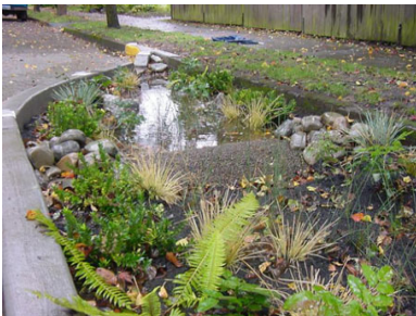
Rain garden within a curb extension.
