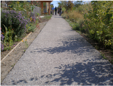
Sidewalk constructed of pervious concrete.
