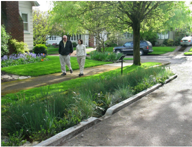
Curb extension with rain garden.
