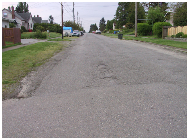
A poorly defined street edge and deteriorated pavement on S Monroe St.
