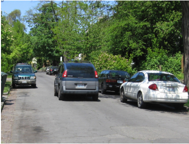
A 28 foot street with parking on both sides provides clearance for one vehicle in the drive lane, requiring queuing when there are two vehicles approaching one another.
